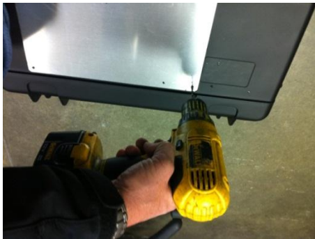
Use holes on plate as drilling template
